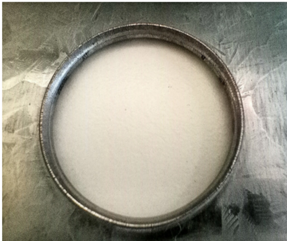
Smooth edges of the Rondo Steel Stud bellmouth service hole
